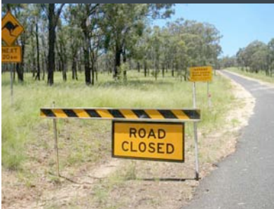
Due to flood damage many rural roads remained closed
