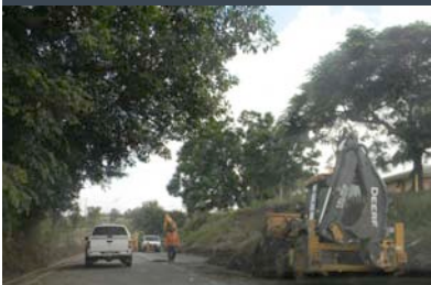
Road repairs will continue for many months
