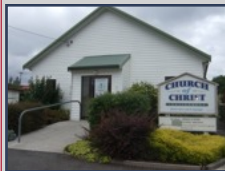
Ulverstone Church of Christ Building
